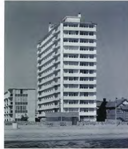
Edgewater Towers, Marine Parade, St Kilda, Vic. (1960). Architect: Mordechai Benshemesh. Photograph: Lyle Fowler, 1962. Source: Harold Paynting Collection, State Library of Vic.
