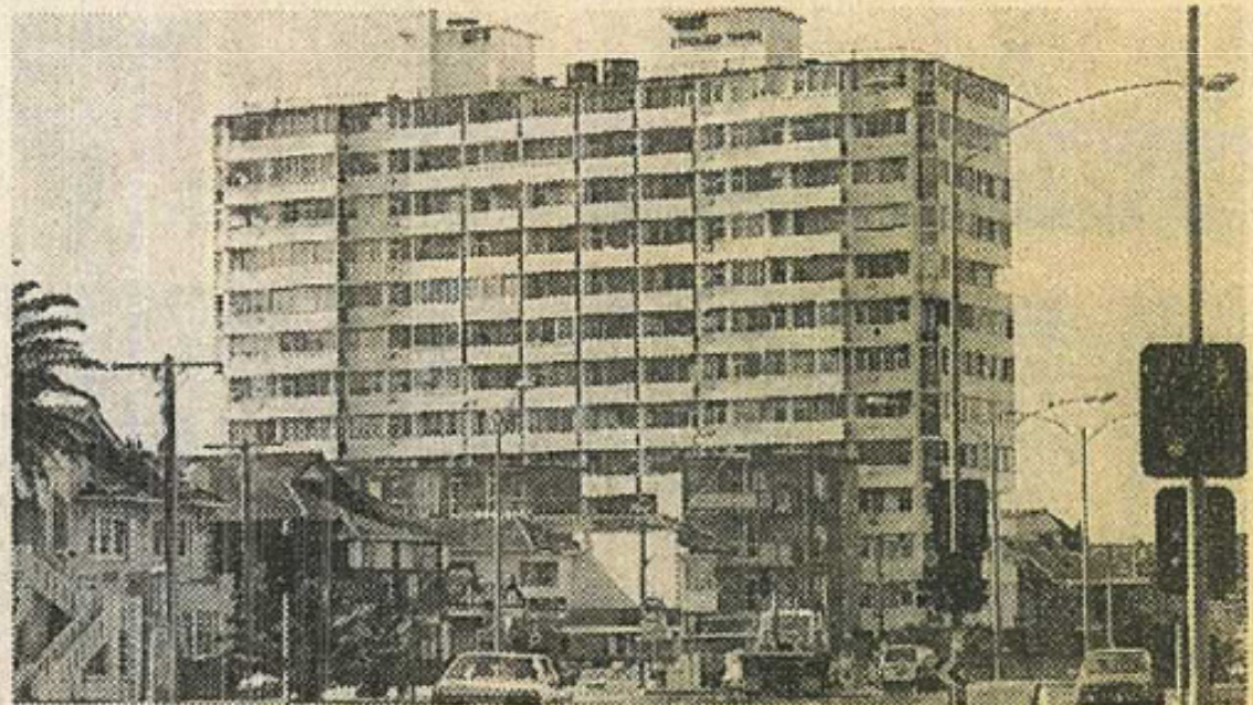
The Edgewater Towers ... a test case for fire safety
