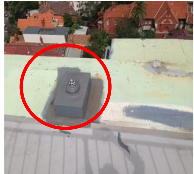
Seven sewer stack vents repaired.
