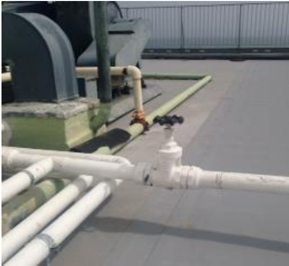
Isolation valve hand wheels rotated to fit below pavers.
