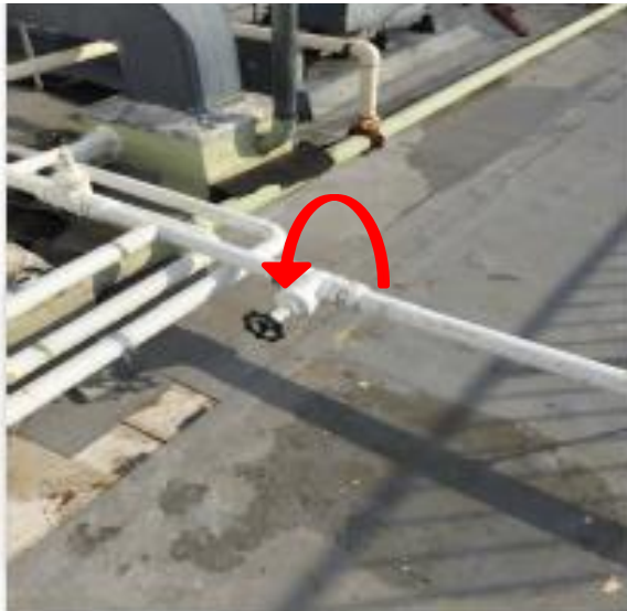
Isolation valve hand wheels rotated to fit below pavers.
