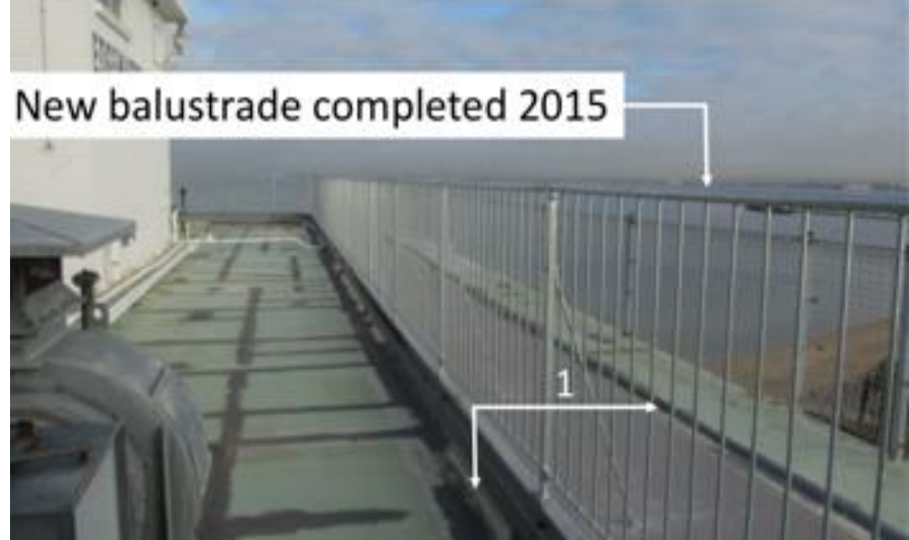
2015 Balustrade installation. First stage of Butynol waterproof membrane.
