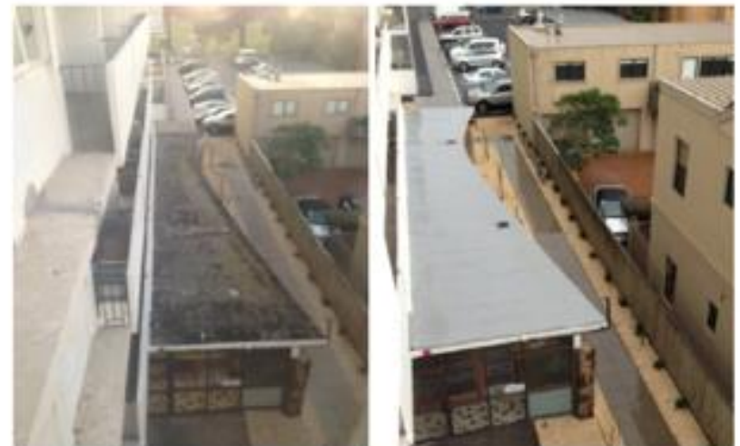
2013 Proposed rooftop Butynol waterproof membrane system prototyped on lobby roof.
