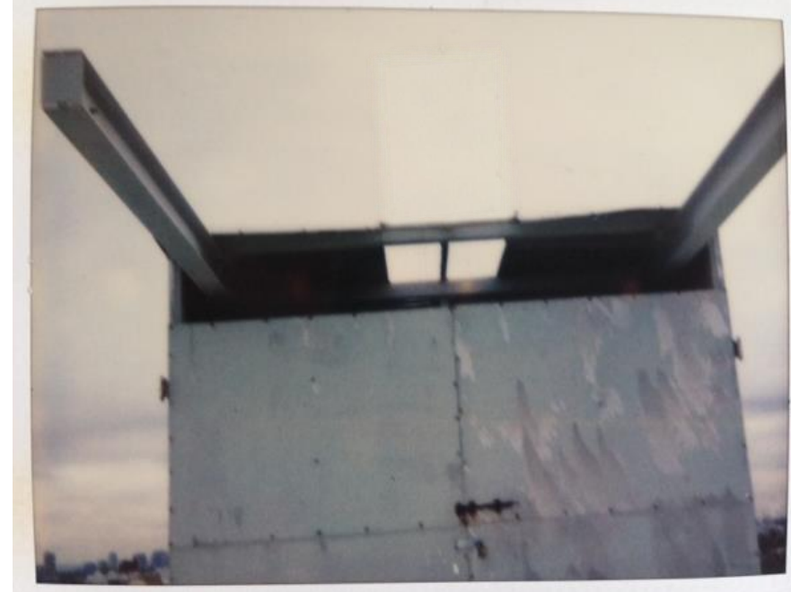
2013 Redundant Building Maintenance Unit (BMU) removed.
