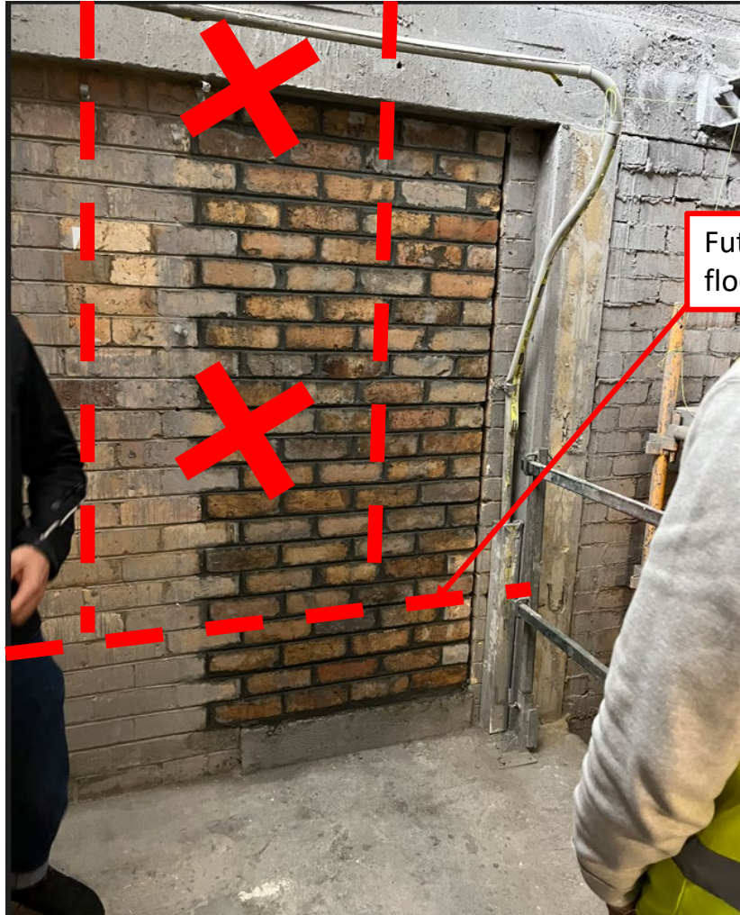
14th December 2022 – Old doorway bricked in prior to concrete beam removal and new doorway.
