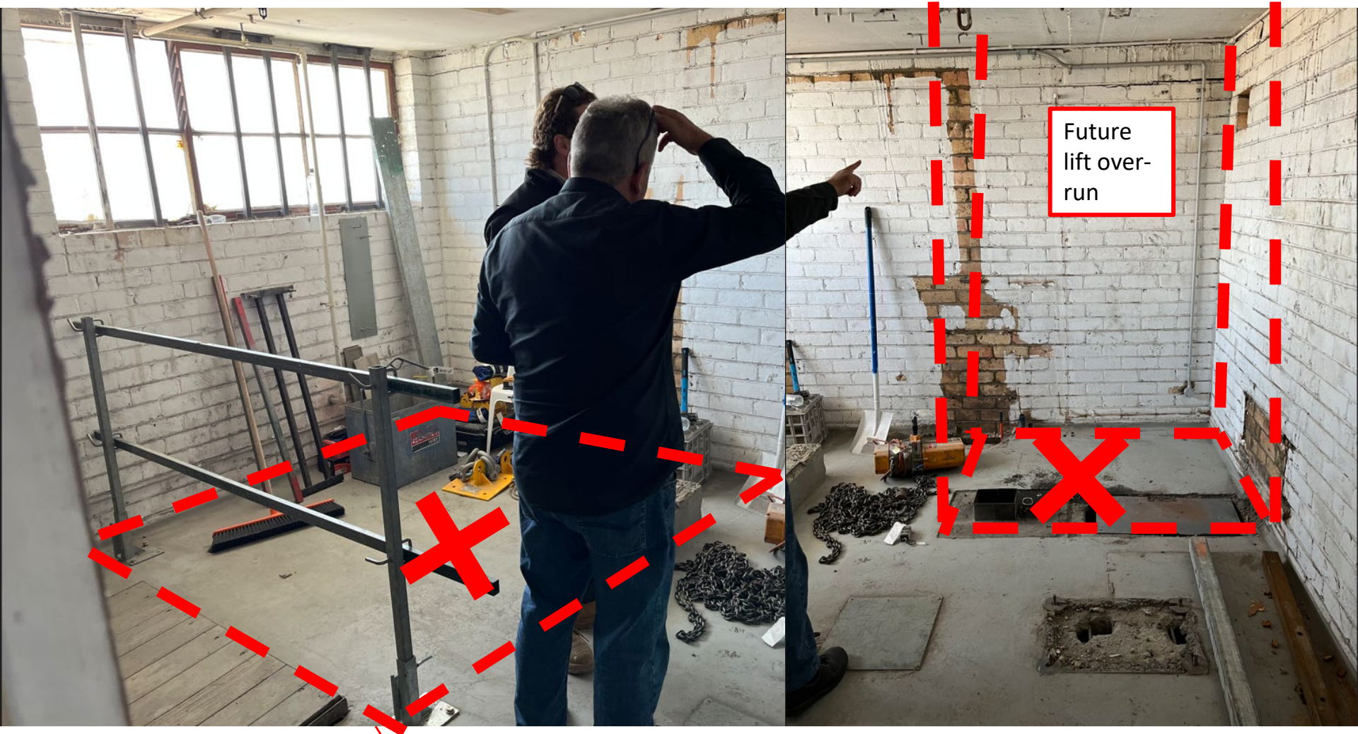
29 th November 2022 – Old Lift Motor Room and machinery removed. Floor slab to be demolished for new lift shaft.
