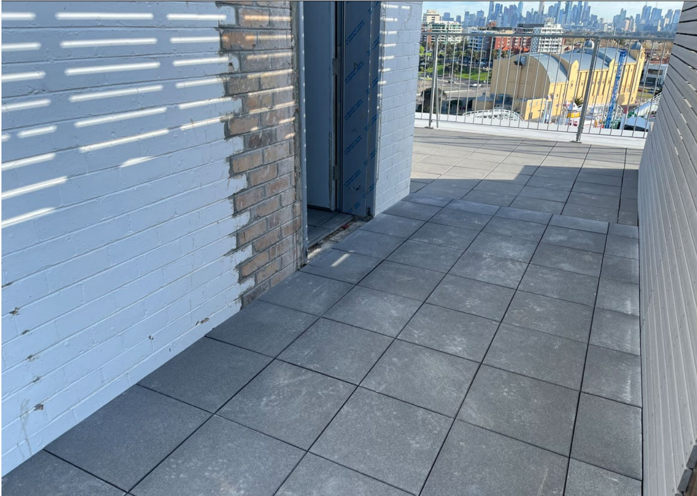
12th September 2023 – New flat floor access to rooftop terrace.
