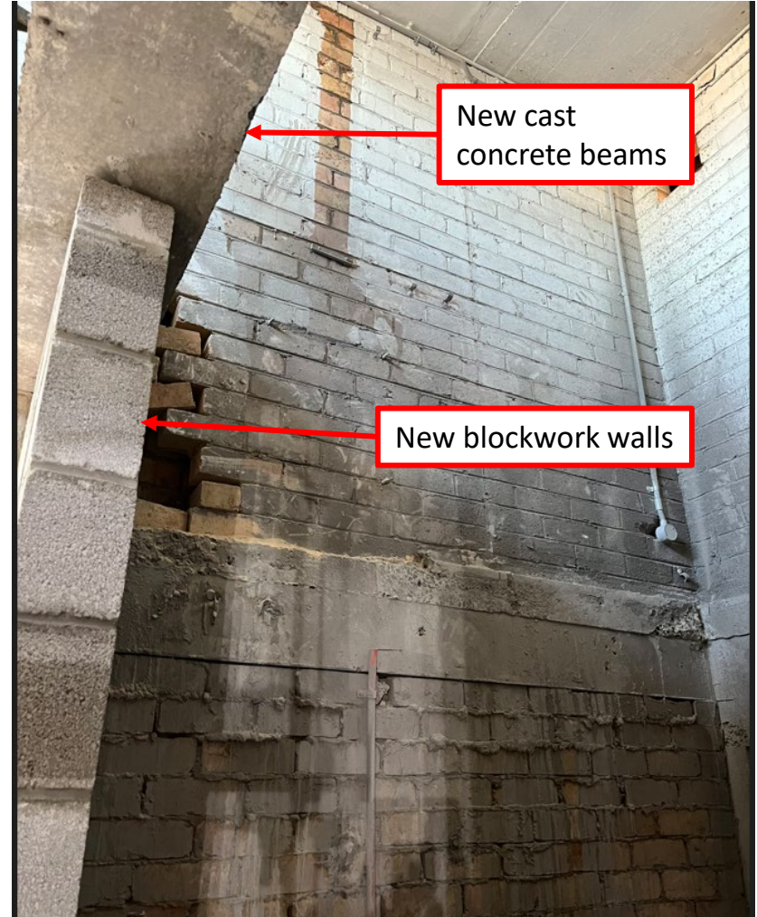
22 nd February 2023 – New structural steelwork. New concrete structure and blockwork lift shaft wall.
